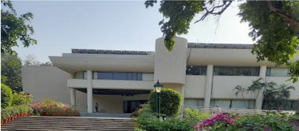
Fig.1: Building Location of the Prime Minister's Museum and Library, New Delhi
